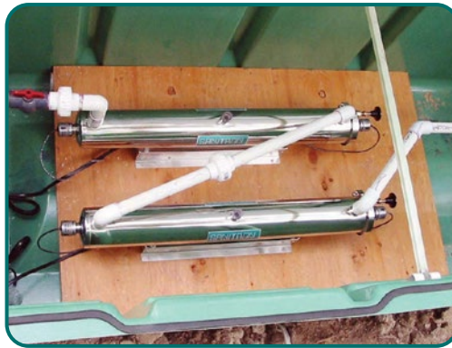
Outside Pond Installation
