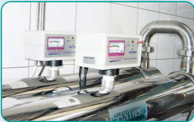
Beverage Processing Plant, Uganda
