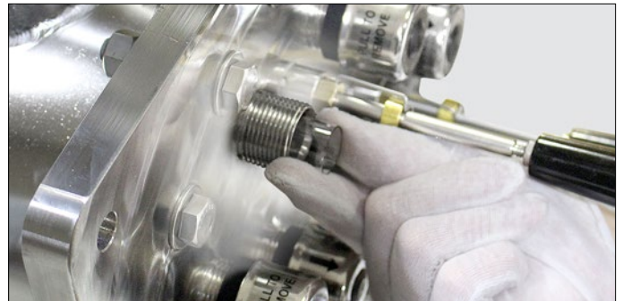
Step 8: With One Person Supporting Quartz Sleeve with a Finger, Have Other Person Carefully Remove Quartz Sleeve
