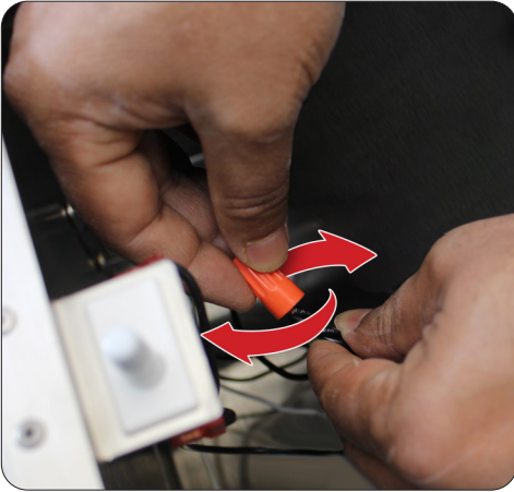
Figure 4 – Reinstall Wire Nuts
